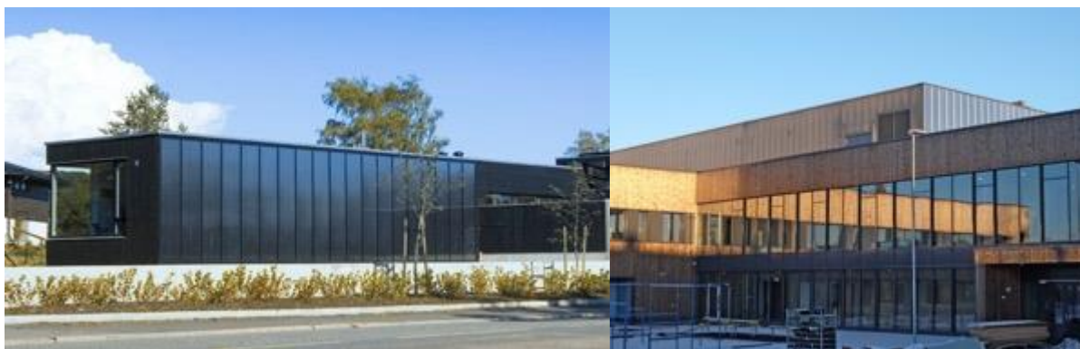
FIGURE 18 FACADE INTEGRATED AVENTASOLAR SOLAR THERMAL COLLECTORS. IMAGE SOURCE: [35]
