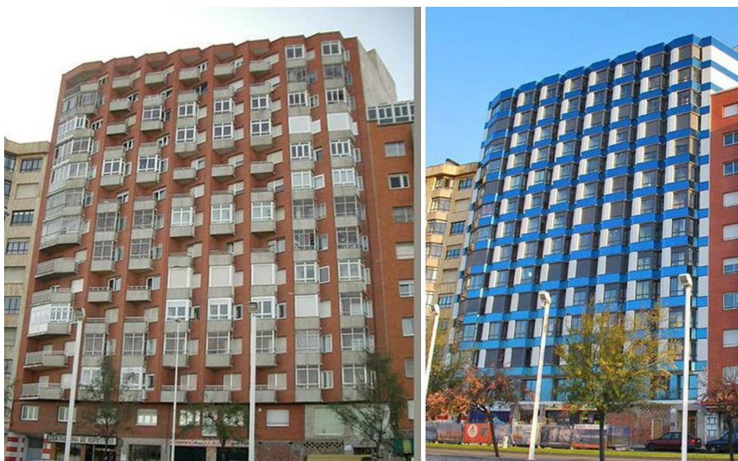
FIGURE 30 DOUBLE SKIN FAÇADE WITH ORIGINALLY LOAD-BEARING FAÇADE. IMAGE SOURCE: [72]
