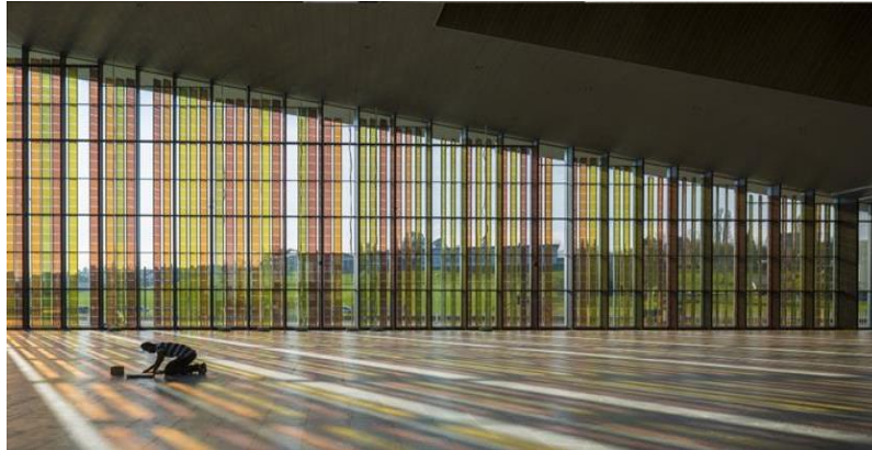
FIGURE 16 SEMI-TRANSPARENT BUILDING INTEGRATED PHOTOVOLTAIC AT THE ÉCOLE POLYTECHNIQUE FÉDÉRALE DE LAUSANNE. IMAGE SOURCE: [35]
